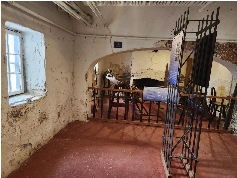
Another view of the "tank", now interpreted as the "workshop". When the Jail closed in 1965, the road gang was kept there.
